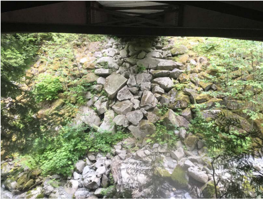
Right Bank Abutment when facing downstream
