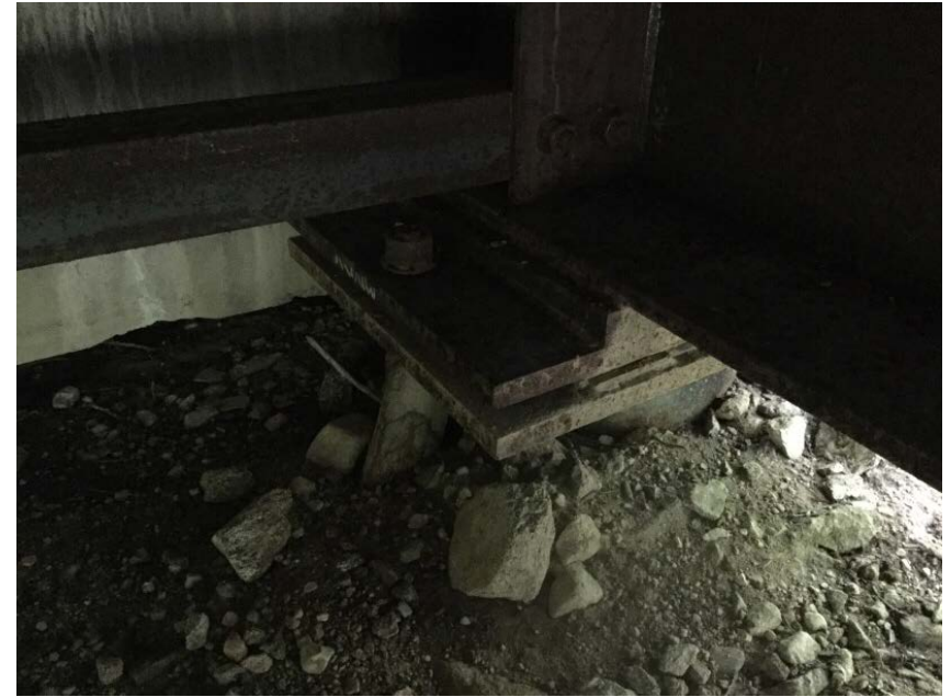
Shim plates for bridge grade, typical
