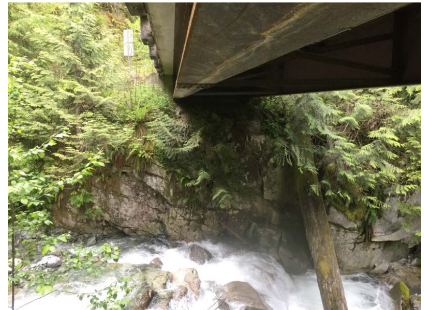
Left Bank Abutment when facing downstream
